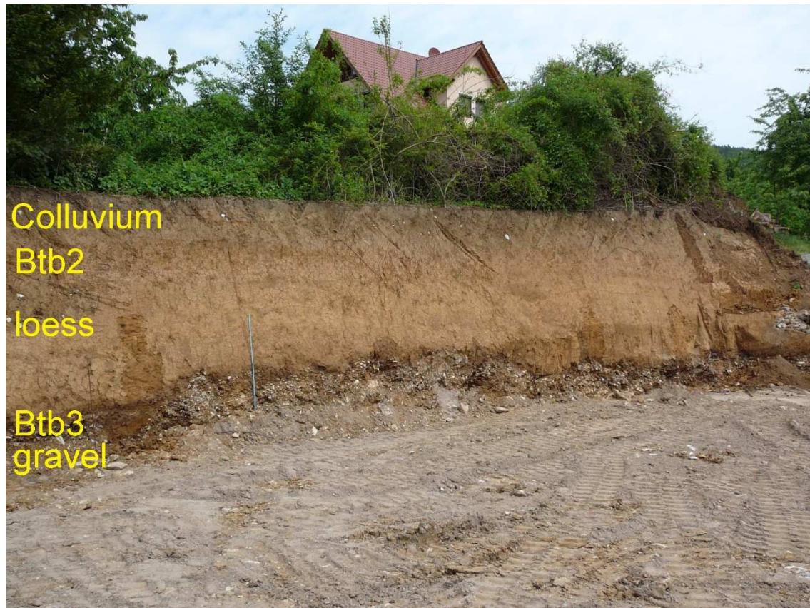
Figure 3: Wannbach site 1. Construction pit of house number 71. Blue meter stick 1.20 m. Note the irregular top line (unconformity) of the gravel bed (penultimate glacial). Its red brown topping flood loam and soil (Btb3) is thicker preserved only in some hollows in the top of the gravel (last interglacial complex). A following thick layer of loess loam (Weichselian) is topped by the fossil early Holocene soil (Btb2) and followed by a grey colluvial humic sequence that embraces an ABtb1 horizon. Photo: W. SCHIRMER 14.05.2007.
